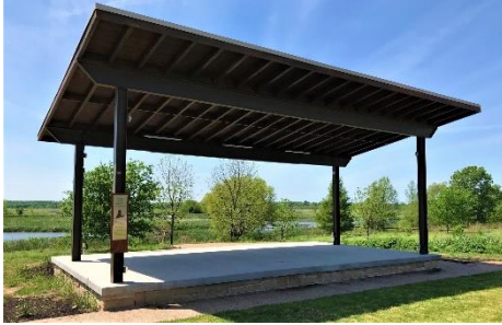
LIGHTED PAVILION WITH ELECTRICITY
