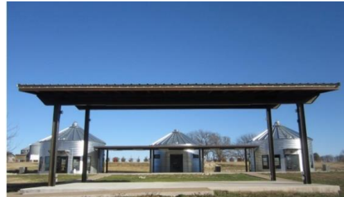
VIEW OF SILOS AND COVERED TERRACE FROM PAVILION
