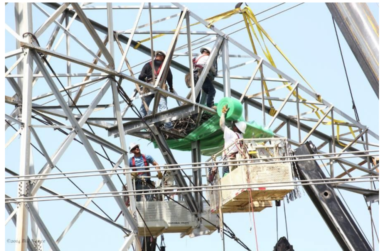
Nest is prepared for relocation to a safe new tower structure. July 2014.
